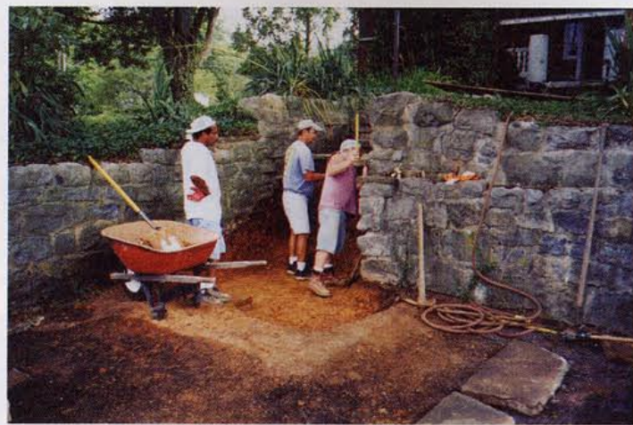
The stone retaining wall and stairs were repaired once the debris was removed.
