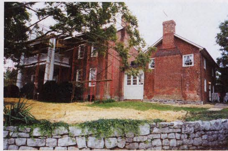
The stone retaining wall and stairs were repaired once the debris was removed.
